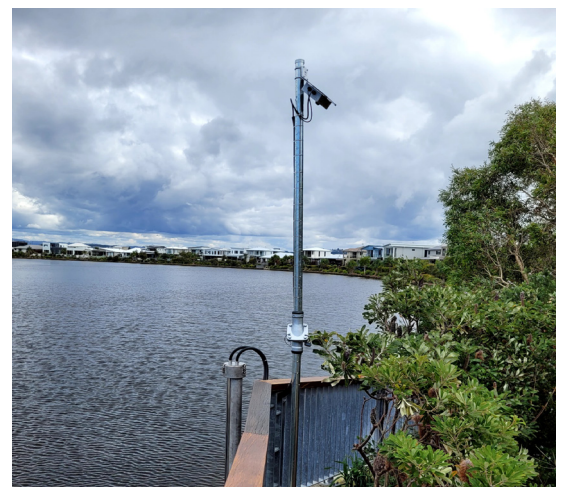
Figure 3. Solar Water Quality Monitoring Station
